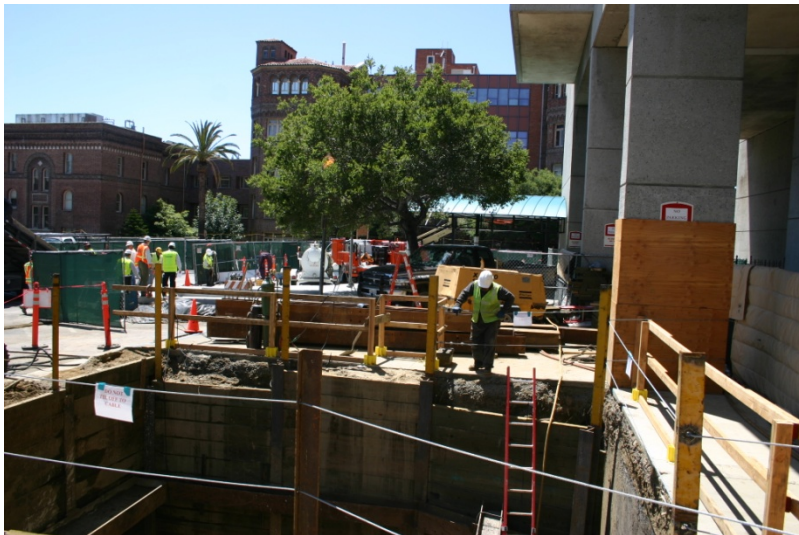
ACCESS PIT TO BUILDING 5 BASEMENT
