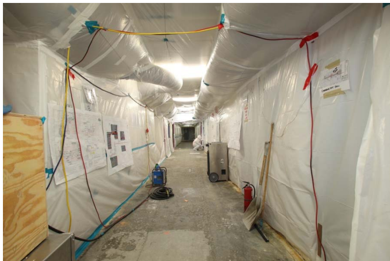
AREA OF WORK INFECTION CONTROL CONTAINMENT
