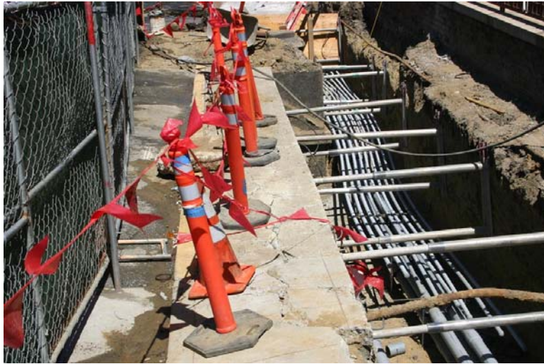
ELECTRICAL DUCTBANK INSTALLATION
