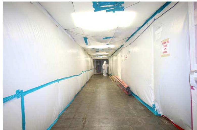
AREA OF WORK INFECTION CONTROL CONTAINMENT
