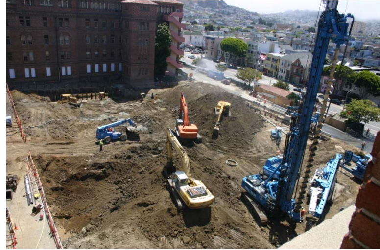
DRILLING RIG OPERATION FOR SHORING
