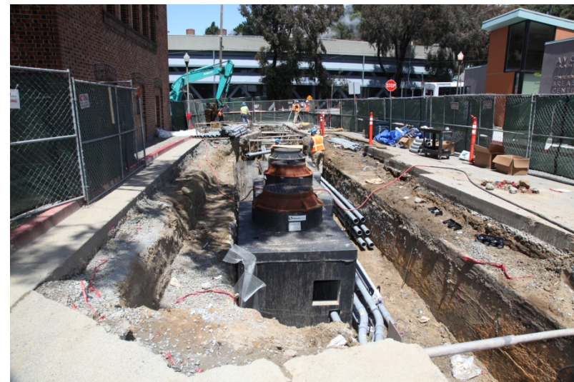
UTILITY VAULT INSTALLATION
