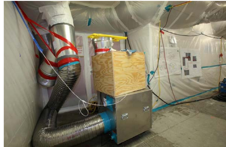
AREA OF WORK NEGATIVE AIR PROVISIONS
