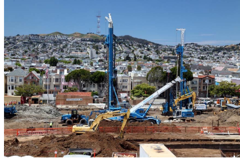
DRILLING RIG OPERATION FOR SHORING
