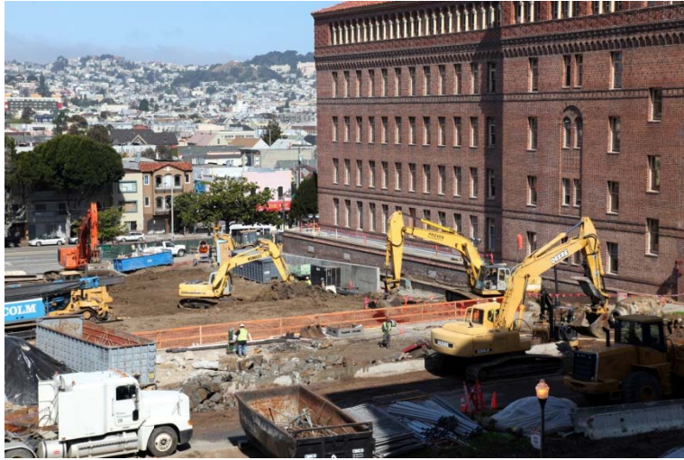
SOIL EXCAVATION AND REMOVAL
