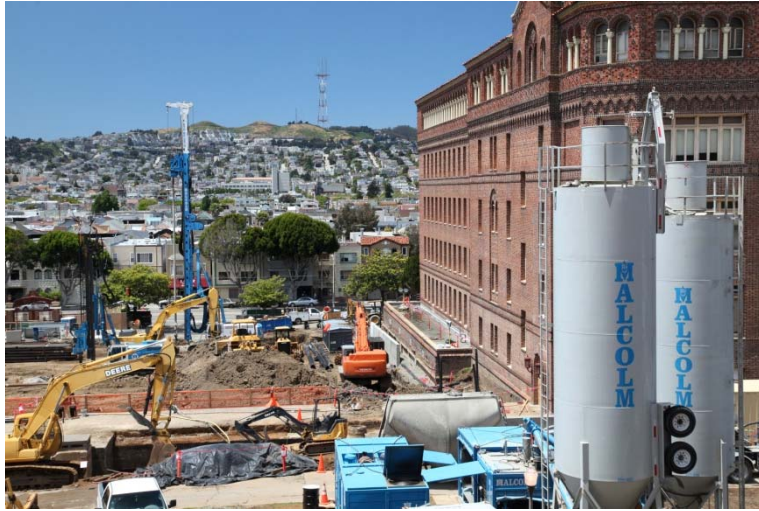
SOIL EXCAVATION AND GROUT PLANT
