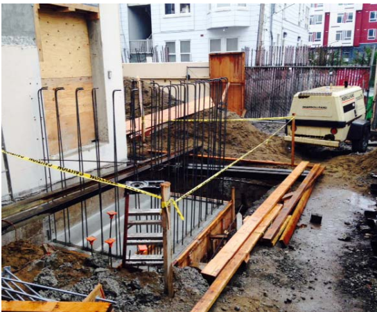
Station 36: Elevator Pit
