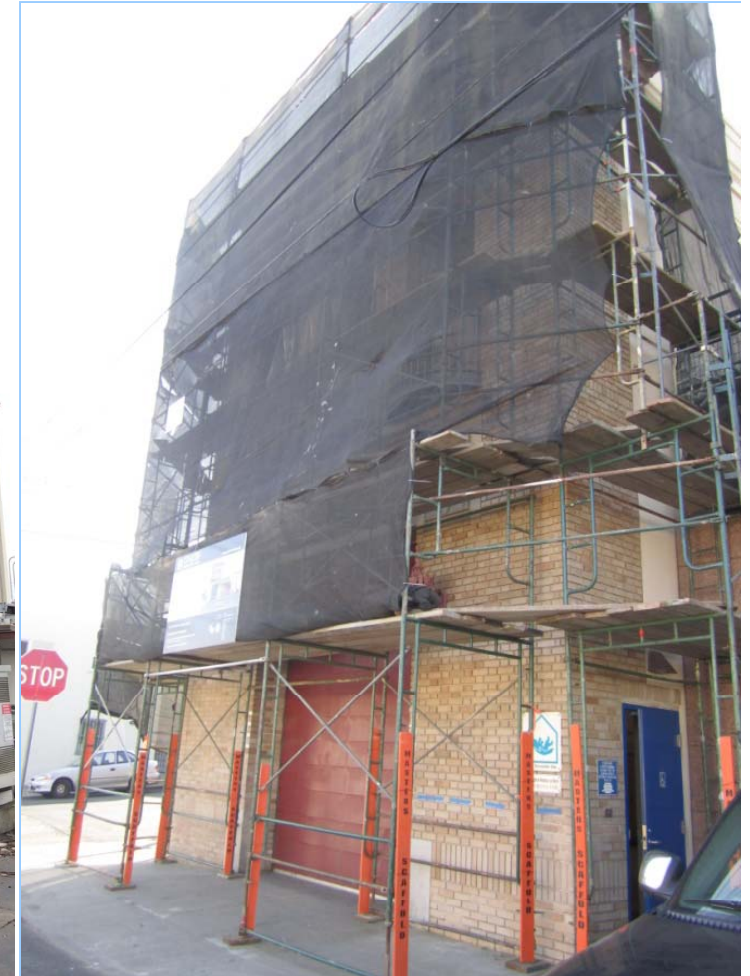
Station 44: Masonry Re-pointing
