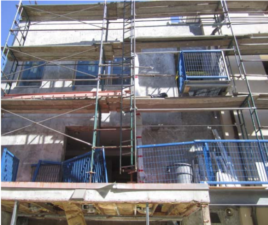
Station 44: New windows installation
