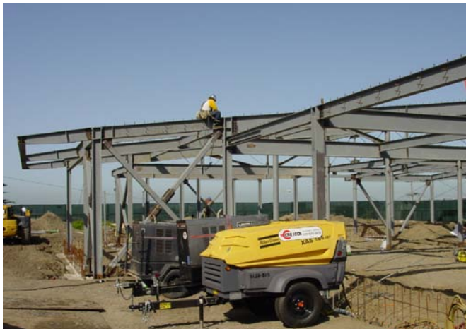
Ortega Branch Library – Steel Framing Work Slated to Open Spring 2011
