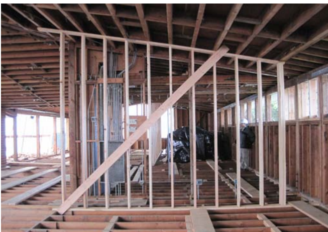
Merced Branch Library – Staff Workroom Wall Slated to Open Winter 2011
