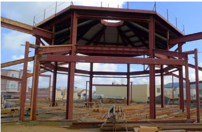
Visitation Valley Branch Library – Southwest View Slated to Open Winter 2010
