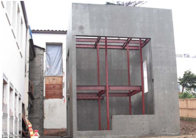
Anza Branch Library - Elevator Tower Slated to Open Winter 2011
