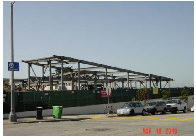
Ortega Branch Library – Steel Framing Slated to Open Spring 2011
