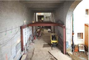
Remodel of the existing Hospital began in June 2007. This work continues in phases in order to minimize the impacts to the operating Hospital. Work in the last quarter included preparation of the underslab utilities for the new restrooms supporting Simon Auditorium and beams to support the new floor level at the mezzanine (level 2). The photograph on the lower right above depicts the initial installation of structural steel to create the connecting corridors for levels one and two.
