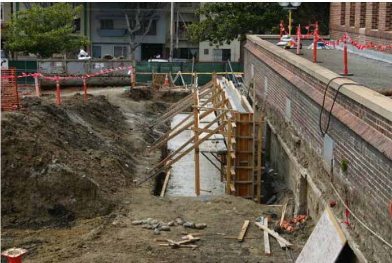
NEW CONCRETE RETAINING WALL
