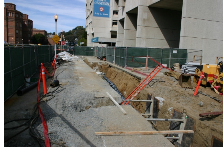
NEW WATER PIPE TRENCHING TO EXISTING HOSPITAL
