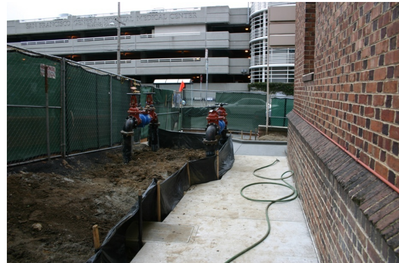
NEW WATER SERVICE & ACCESSIBLE PATH TO SIDEWALK
