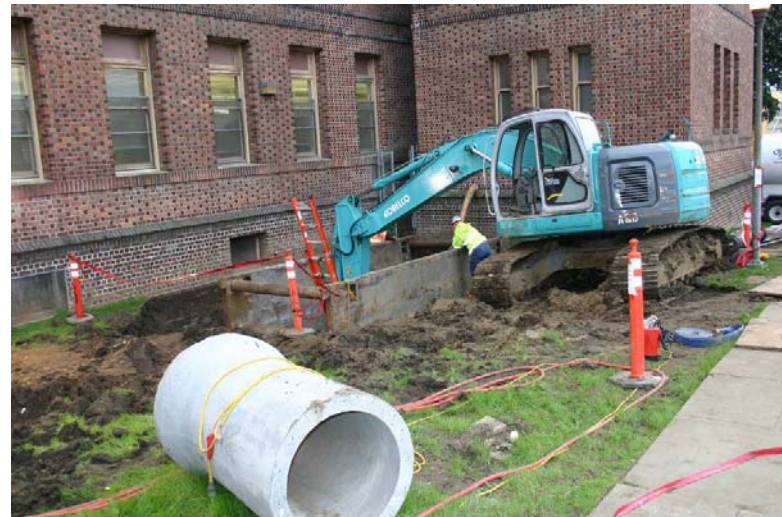
JACK BORING UTILITY LINES UNDER BLD'G 30 TOWER
