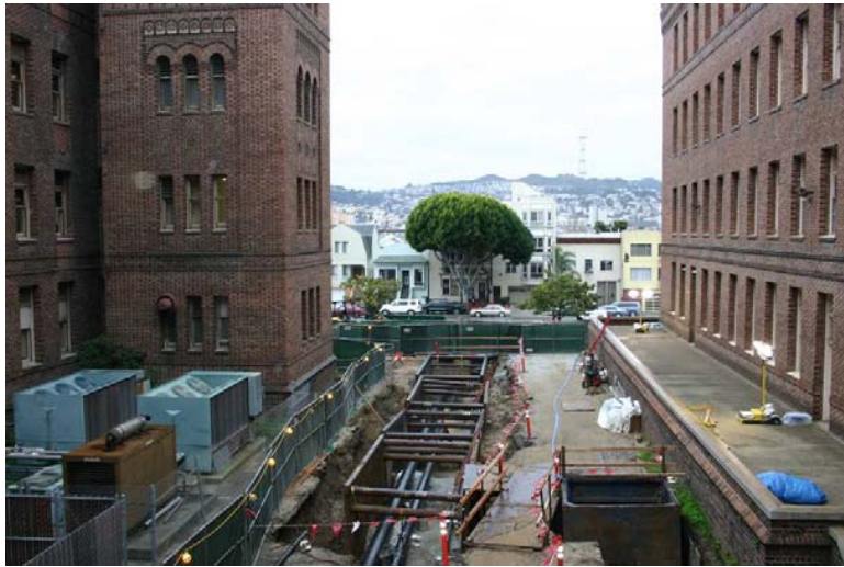
NEW STEAM PIPING AND VAULTS
